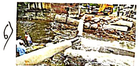
Leakage from sewer Lines
